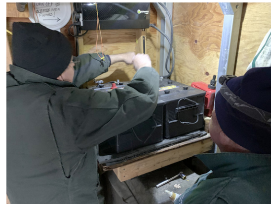
Pete Sarvas methodically connects the new batteries into the system. Everyone was happy to see the volt meters light up when the last wire was attached.
